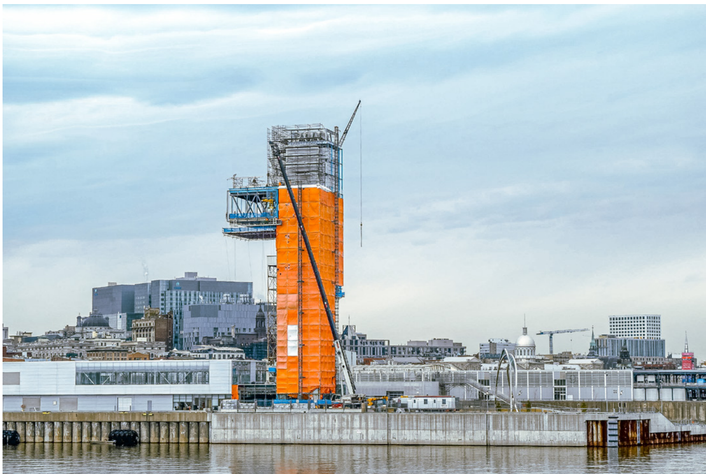
Heavydrive Glasmontage am Tour du Grand Quai in Montréal QC (Kanada)
